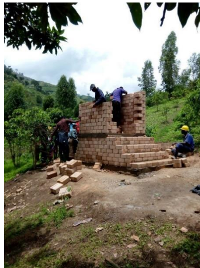
© Gaetan Stassart Construction of an Ecosan latrine.
